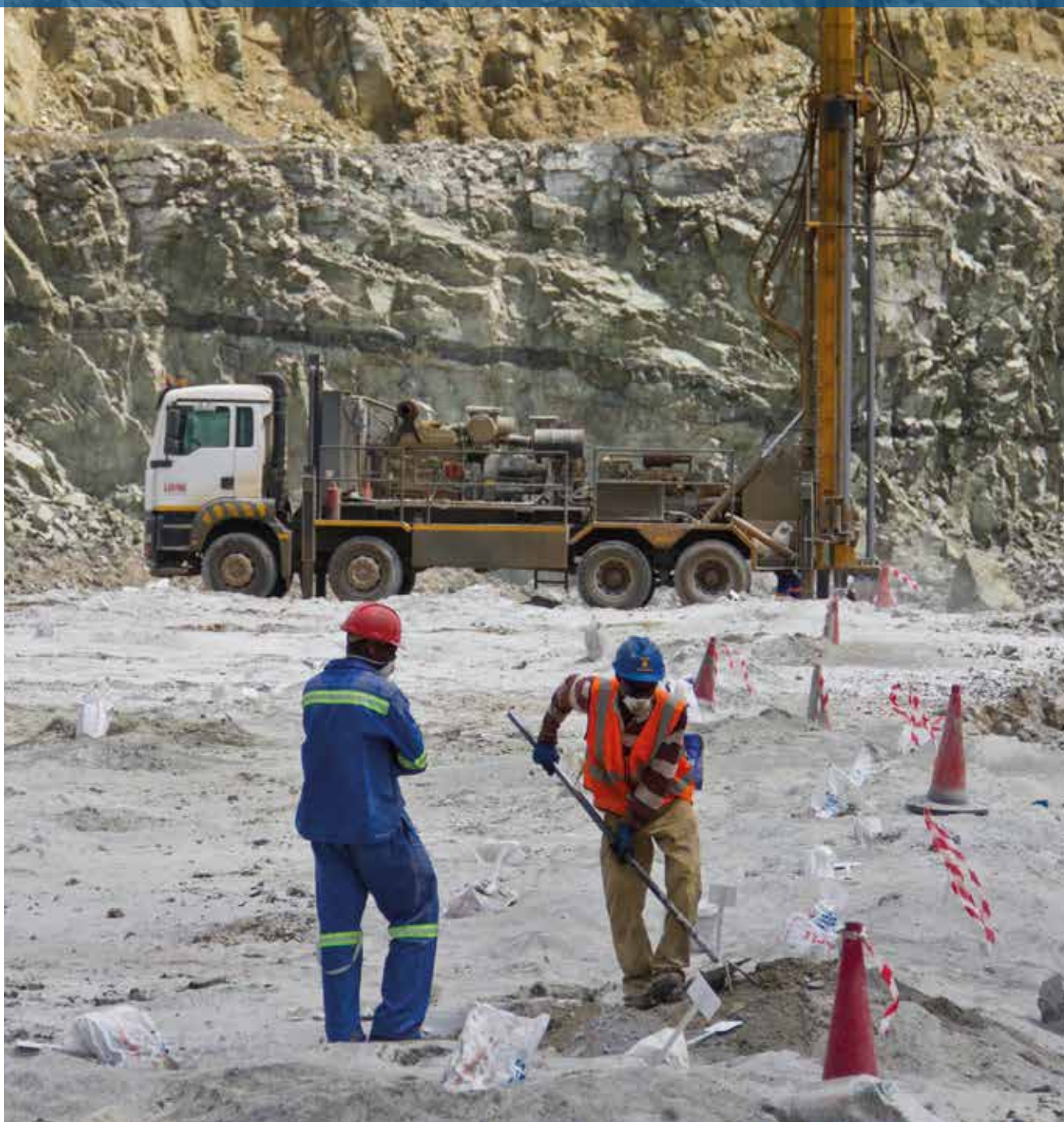
Production drilling and blast hole preparation at the Pilanesberg Platinum Mine.
